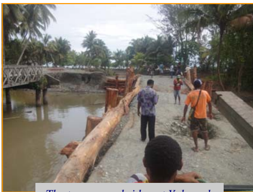
The temporary bridge at Yakamul.
